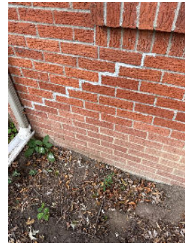
Repair observed on the southeast corner
