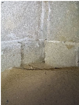
Separation in the block on the southwest corner
