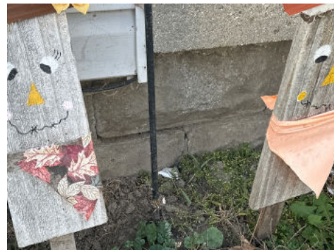
Cracked and loose mortar under front porch
