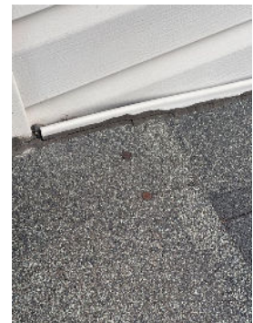
Unsealed fasteners
