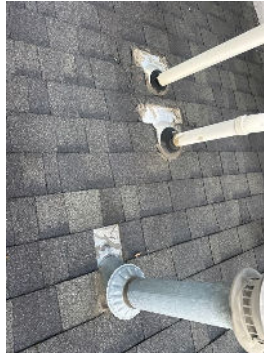
Temporary repairs observed at roof penetrations
