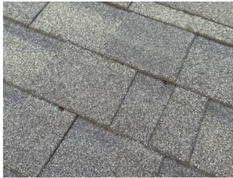
Low nails and granule loss observed
