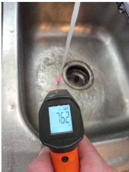
Warm Water Temperature First Floor.
