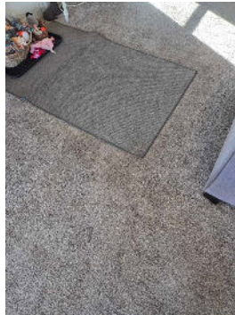
Stained/ worn flooring observed
