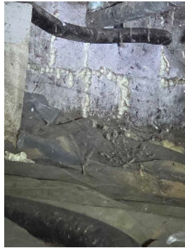
Spray foam repair on north wall
