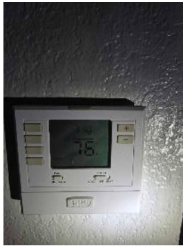
Before Testing Temperature.
