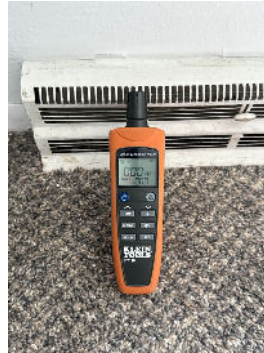
Carbon Monoxide Reading Unit 1.
