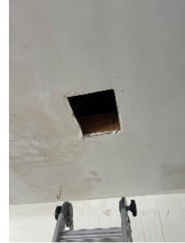
Access Point for garage attic. Very limited access to due opening size.
