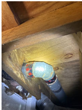
Mold like substance observed along the south side subfloor
