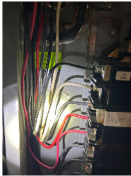
Unmarked neutral being used as a hot feed
