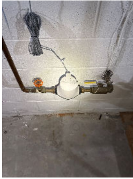
Current Condition Unit 1
