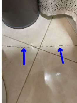
Cracked tiles observed.
