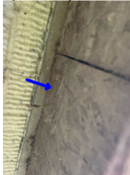
Exposed wood on the east end kickout
