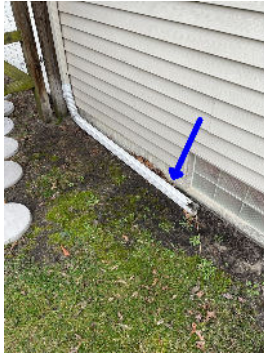
The downspout on the northeast corner of the home should not discharge against the house
