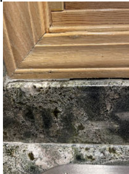
Backsplash needs to be sealed to the window.
