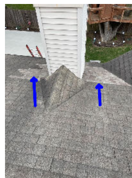
Large repair observed around the chimney
