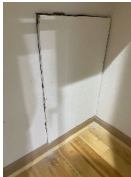
Access panel is loosely attached.
