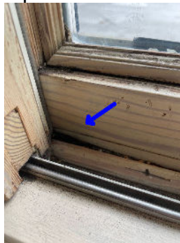
Stationary panel on the patio door is rotted.
