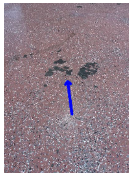
There are a few smaller damaged spots of finish epoxy
