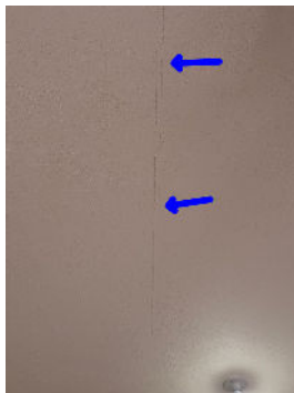
Common tape seam cracks noted
