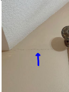
Settling crack.
