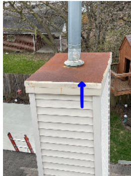
The metal cap is heavily rusted
