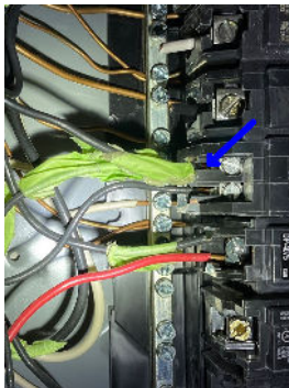
Double tapped breaker observed
