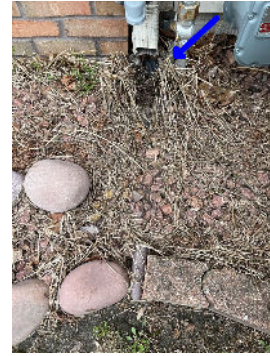
Missing downspout extension on the southwest corner
