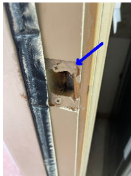
Missing strike plate observed
