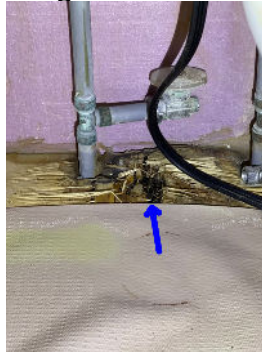
Sink base cabinet is damaged.
