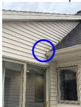
Missing kickout flashing on the east end
