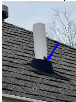
Multiple torn soil stack boots
