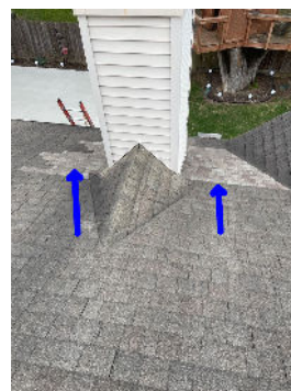
Large repair observed around the chimney
