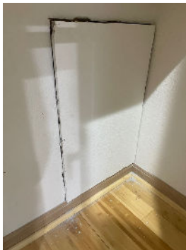
Access panel is loosely attached.
