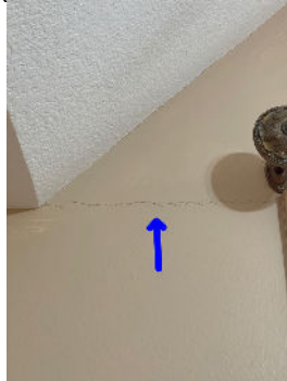
Settling crack.
