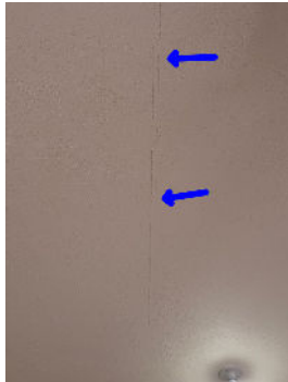
Common tape seam cracks noted
