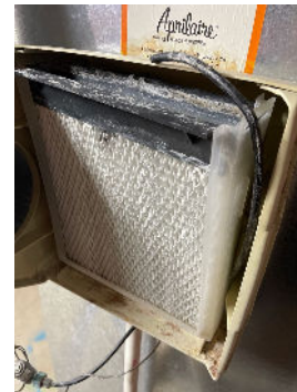
Damaged humidifier internals observed
