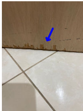
Bottom of the door is delaminating.
