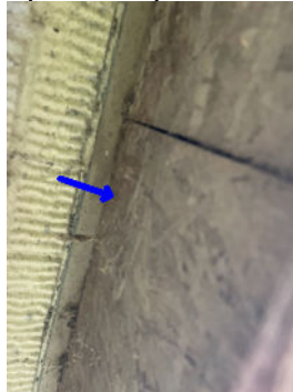
Exposed wood on the east end kickout
