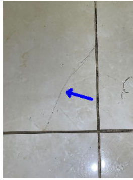
Cracked tiles observed in several spots.
