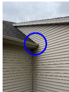
Missing kickout flashing on the southeast corner
