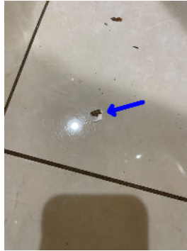
Damaged tile observed.
