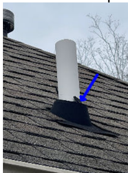
Multiple torn soil stack boots
