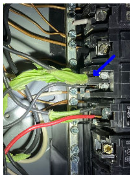
Double tapped breaker observed
