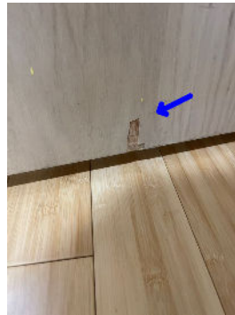
Door is delaminated.
